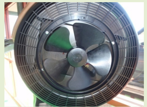
The fan draws hot air from the roof of the house
